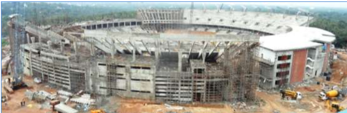
Status of the Greenfield Stadium, Karyavattom as on 1 st November 2014
