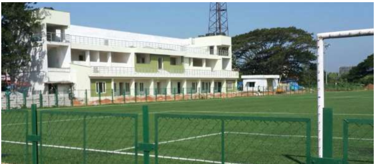
New pavilion at Corporation Stadium, Thrissur
